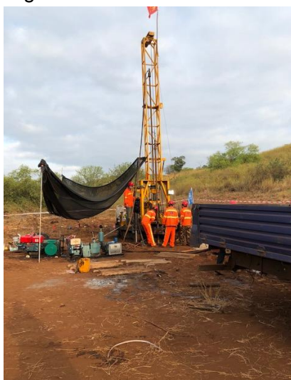
Image 1: Drilling rig in operation at CdB
